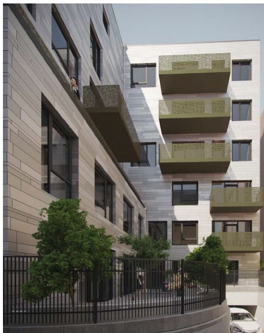
Image of the metal cladding to be used at the rear and for the top storey
